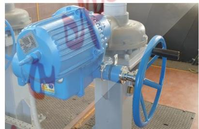
Emergency Kit on DREHMO Electric Actuator
